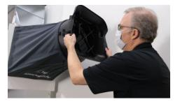
2, Option #2: Capture individual flow reading from every independent return with a passive flow hood. Combine the readings for total flow measurement.
