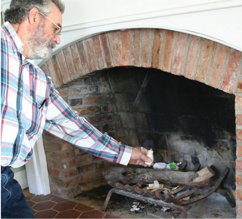
Figure 4. In a depressurized house, air will rush in through any available opening, so combustion appliances need to be shut down during a blower-door test to prevent backdrafting. Here, a smoke puffer indicates that the chimney flue is leaky even with its damper fully closed.
