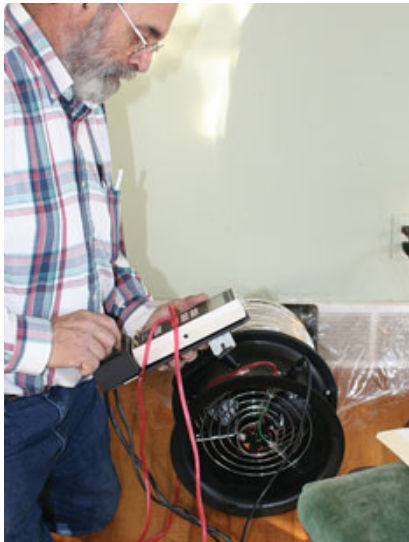
Figure 7. Duct system leakage can be estimated using the “blower-door subtraction method,” but a Duct Blaster test is more accurate. After the supply and return registers are sealed with tape, airflow is directed into the supply plenum, measured at a reference pressure of 25 Pa, and compared with accepted leakage rates.
