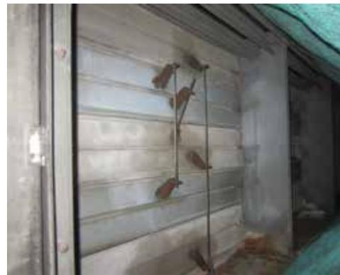
>> During the test, all mechanical dampers are closed and the dampers or terminations of the outside air ducts, exhaust air ducts and exhaust fans were temporarily sealed.
