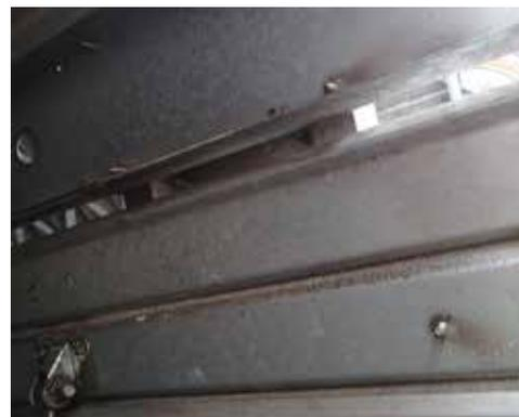
>> With the dampers closed, this RTU revealed an opening for inevitable leakage and air infiltration.
