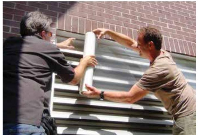
⚡ **Preparing the building by sealing HVAC openings and unsealing them after the test will often be the most time-consuming part of the entire test process.**
