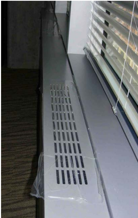
Figure 13: Sealed perimeter linear grilles
