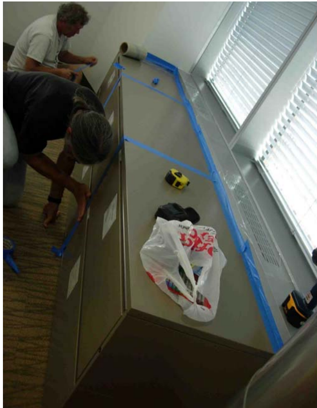
Figure 14: Taping cracks and cabinets at perimeter
