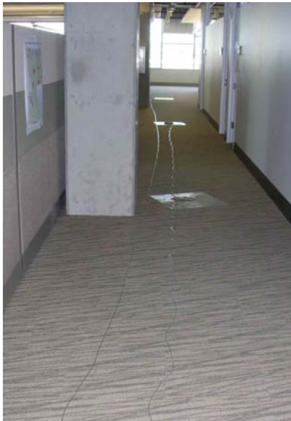
Figure 6: Installation of tubing for plenum pressure measurement
