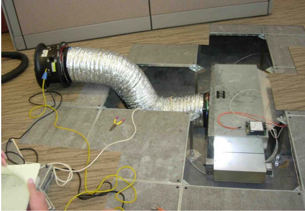
Figure 12: Duct Blaster connected to inlet of fan-coil unit for perimeter system testing
