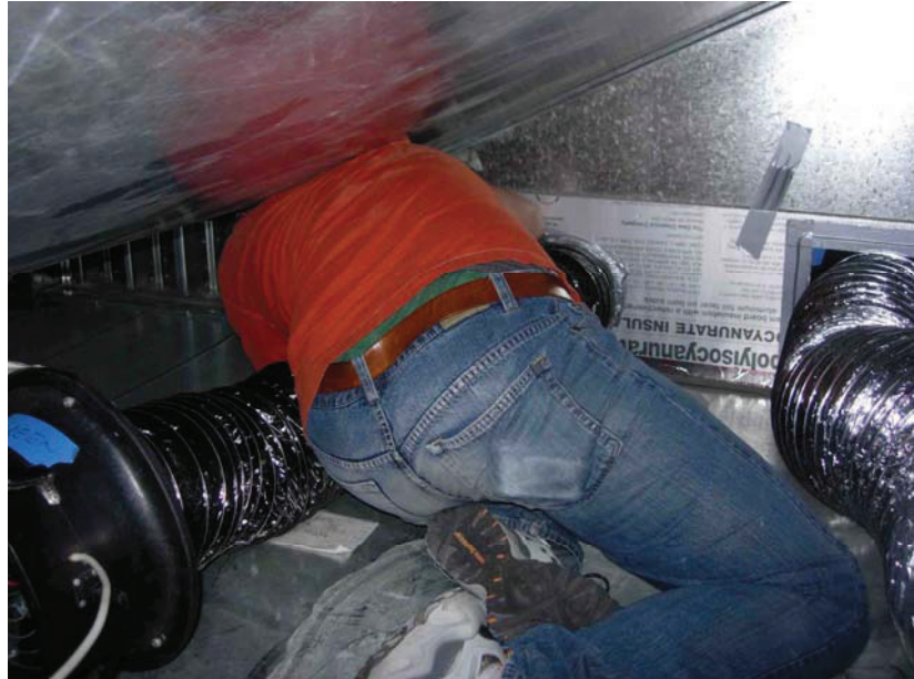
Figure 11: Two Duct Blasters with manifold being installed at entrance to one supply air highway
