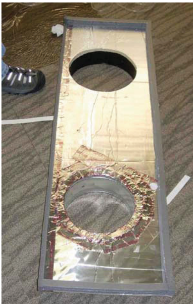
Figure 10: Duct Blaster manifold
