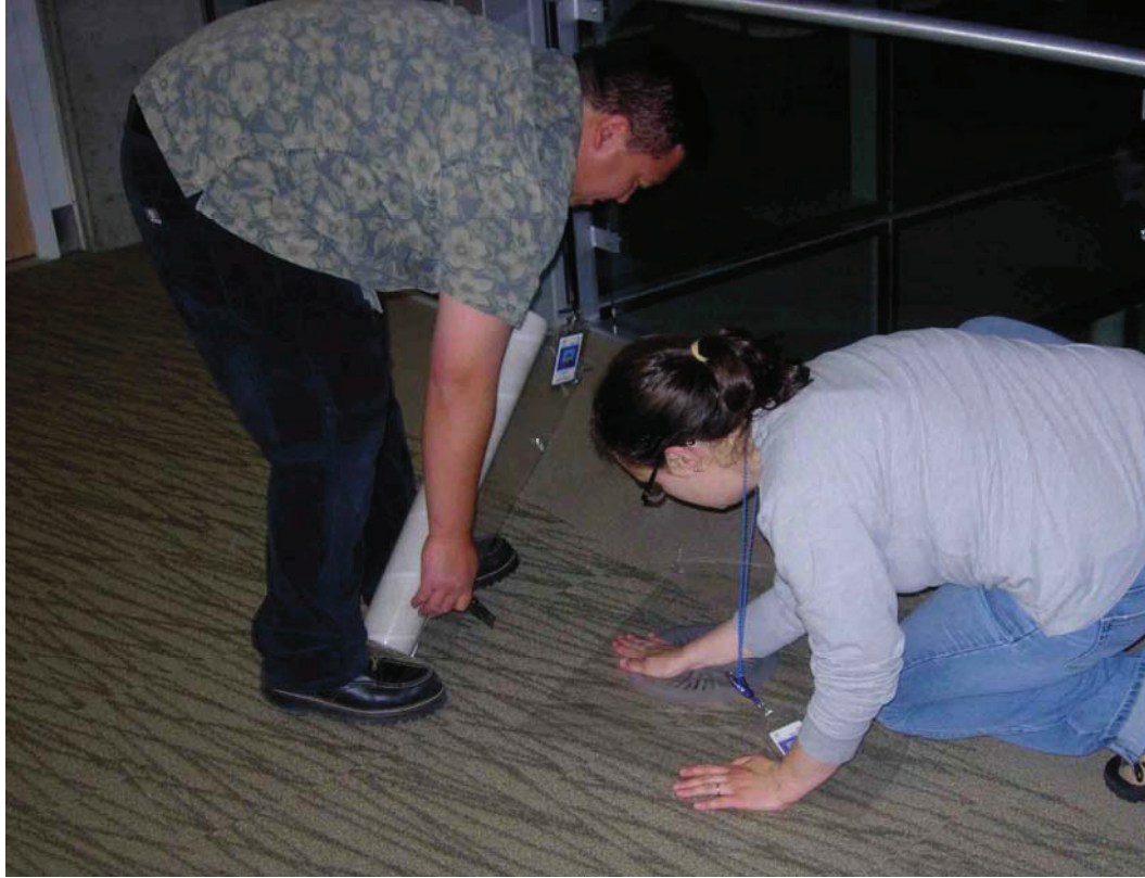
Figure 8: Applying wide “carpet mask” tape over swirl diffuser
