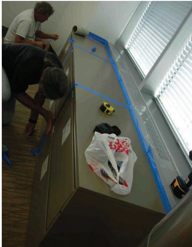
Figure 14: Taping cracks and cabinets at perimeter
