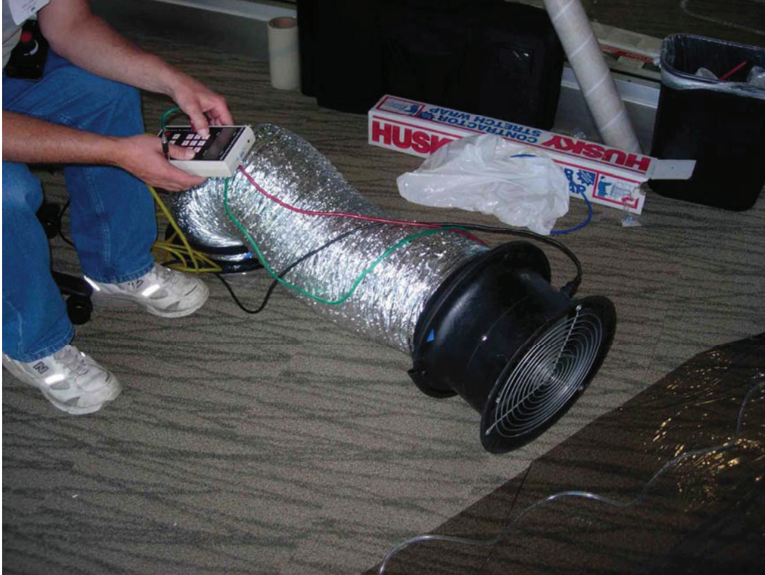
Figure 9: Duct Blaster shown being used as a powered flow hood to measure flow through swirl floor diffuser
