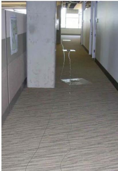
Figure 6: Installation of tubing for plenum pressure measurement
