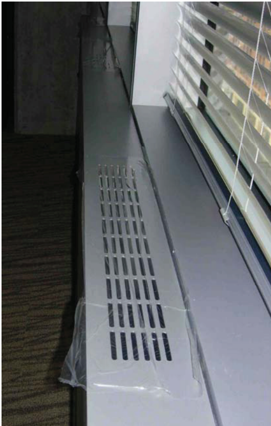
Figure 13: Sealed perimeter linear grilles
