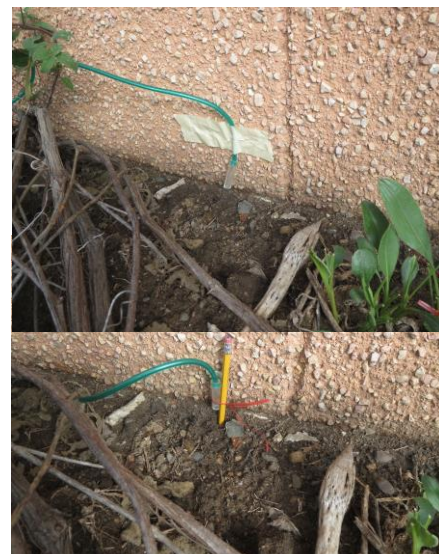
If tape does not stick to the wall, you will need something to hold the tubing up off the ground
