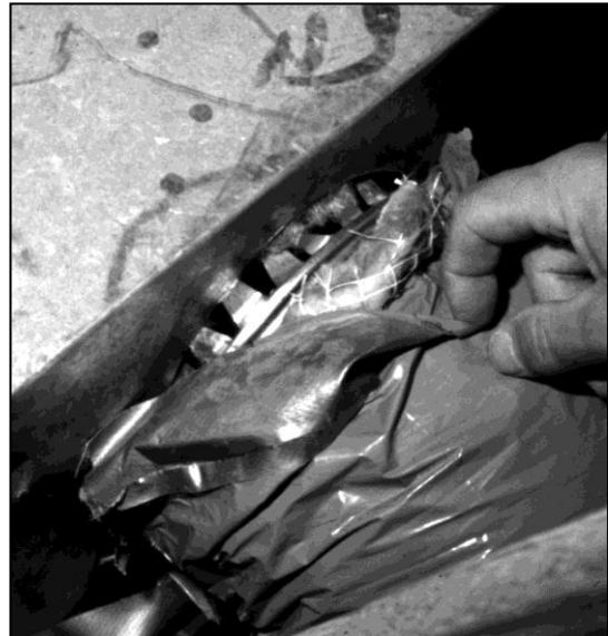
Supply Leak at Take-Off Connection
